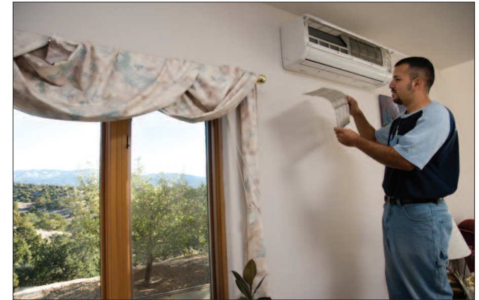
Irvin Marin, service technician, cleaning filters on the indoor Fujitsu pump in Joe Salazar's home
