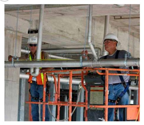
One of the most unique facets of the new facility's construction was the specification for 8,000 lineal feet of stainless steel drainage piping, chosen because of the resilience, durability and thermal characteristics of the material.
