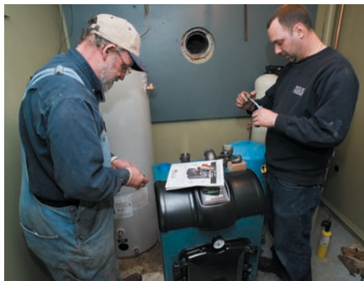
Technicians Spence Walker (l.) and Larry Lawrence begin to assemble supply piping for the new oilfired Burnham MPO boiler
