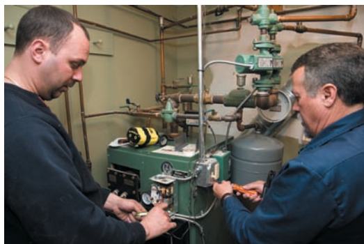
Technician Larry Lawrence (l.) and Yates prepare the original boiler for removal.
