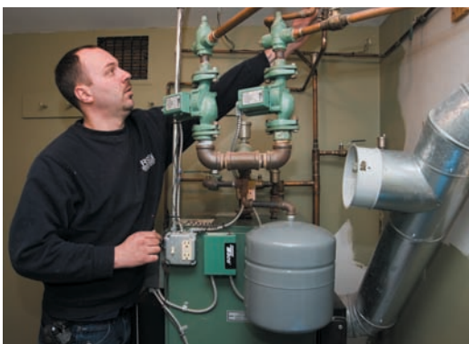
F. W. Behler Technician Larry Lawrence disassembles the near-boiler piping for the original 180 MBH oilfired boiler.
