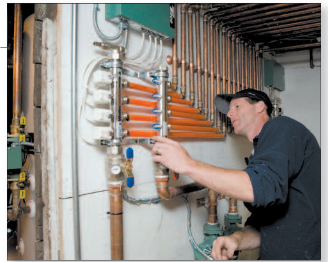
Ken Dunn tweaks flow through the stainless steel manifolds.
