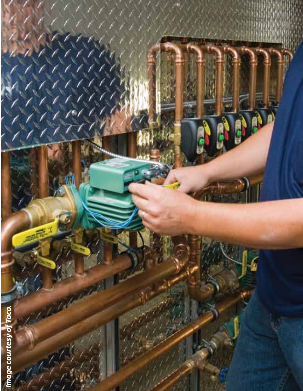
« AA technician completes installation of a variable delta-T pump and zone valves while commissioning a light-commercial radiant-heat system.
