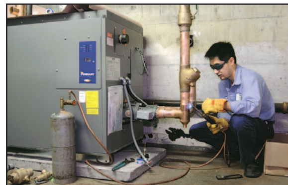
A check valve is installed on the boiler loop piping at the Sherman Street Apartments.
