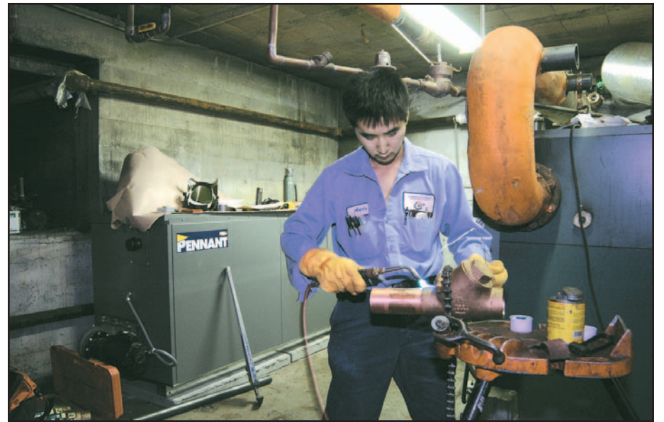
At the Sherman Street Apartment complex, an apprentice solders a 2 1/2" check valve for installation of one Pennant hot water heating boiler.
