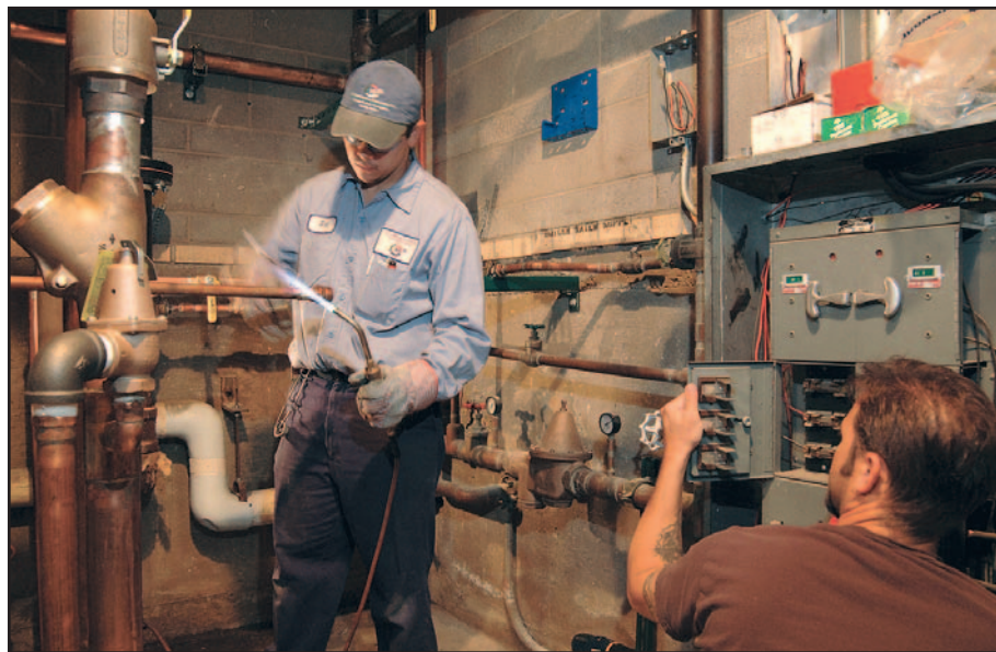
While doing a boiler replacement for a local LDS church, an HVAC apprentice prepares piping for installation of two Pennant hot water heating boilers. Meanwhile, an electrician prepares the wiring for the boilers.
