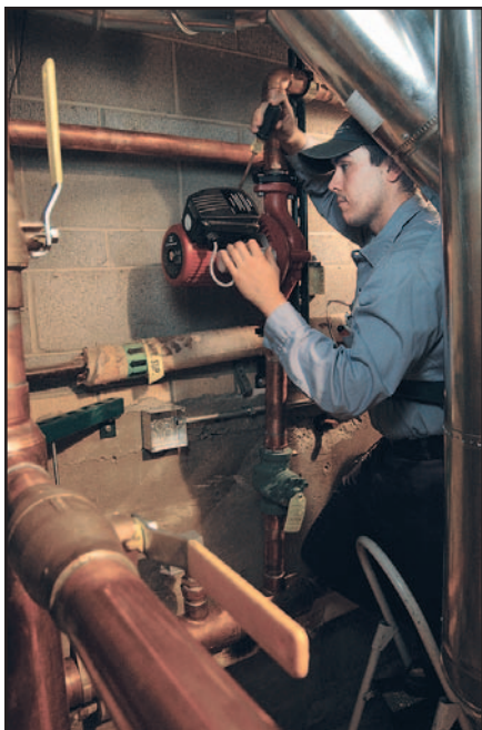
ACA Denver Boiler installed Grundfos 3-speed pumps at a LDS church project.
