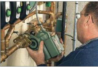
Taco's 008-VDT variable speed,  $\Delta T$  pump varies its speed based on the heating system's Delta T — the water temperature differential between the supply and return piping. Installing one of the pumps in a hydronic system reduces condensate and allows the boiler to hum along at 89% AFUE.
