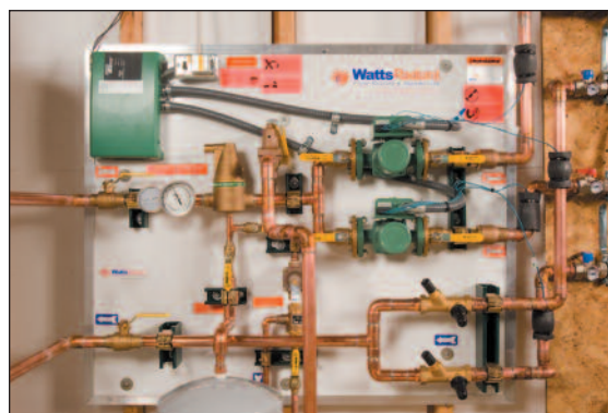
A preassembled, two-zone HydroControl panel from Watts Radiant includes two Taco variable-speed, ΔT pumps, a 4900 Series air separator and a zone control. Watts provided a backflow prevention/auto-feed valve; a two-gallon expansion tank; ISO valves; pressure, temperature and relief valves and balancing valves.
