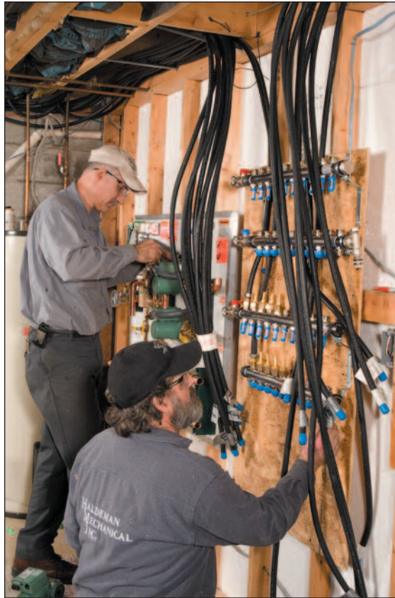
Tavi Nistor (standing) and Bill Aller install the control panel and manifolds for the 2,000 feet of Onix tubing the project required.
