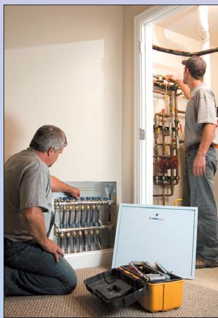
The 39 condos have 2,486 to 2,982 sq. ft. of floor space, with all rooms heated to comfortable levels using radiant floors and zone controls.
