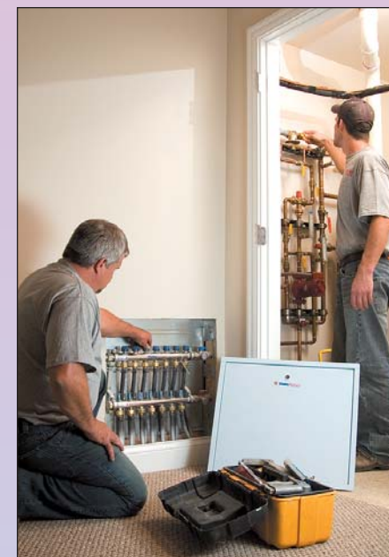
The 39 condos have 2,486 to 2,982 sq. ft. of floor space, with all rooms heated to comfortable levels using radiant floors and zone controls.
