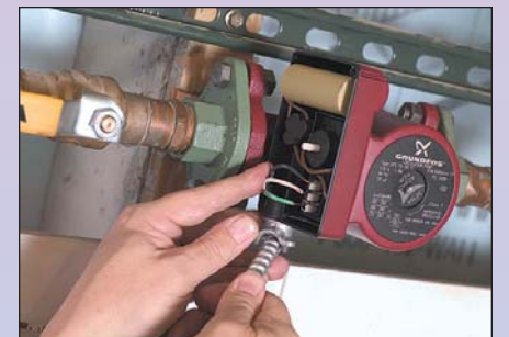
Multi-speed circulators allow contractors to stock far fewer pumps in shop inventory and on trucks.
