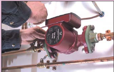
Multiple-speed circulation allows variability of pumps, later system retrofits and provides better system performance.
