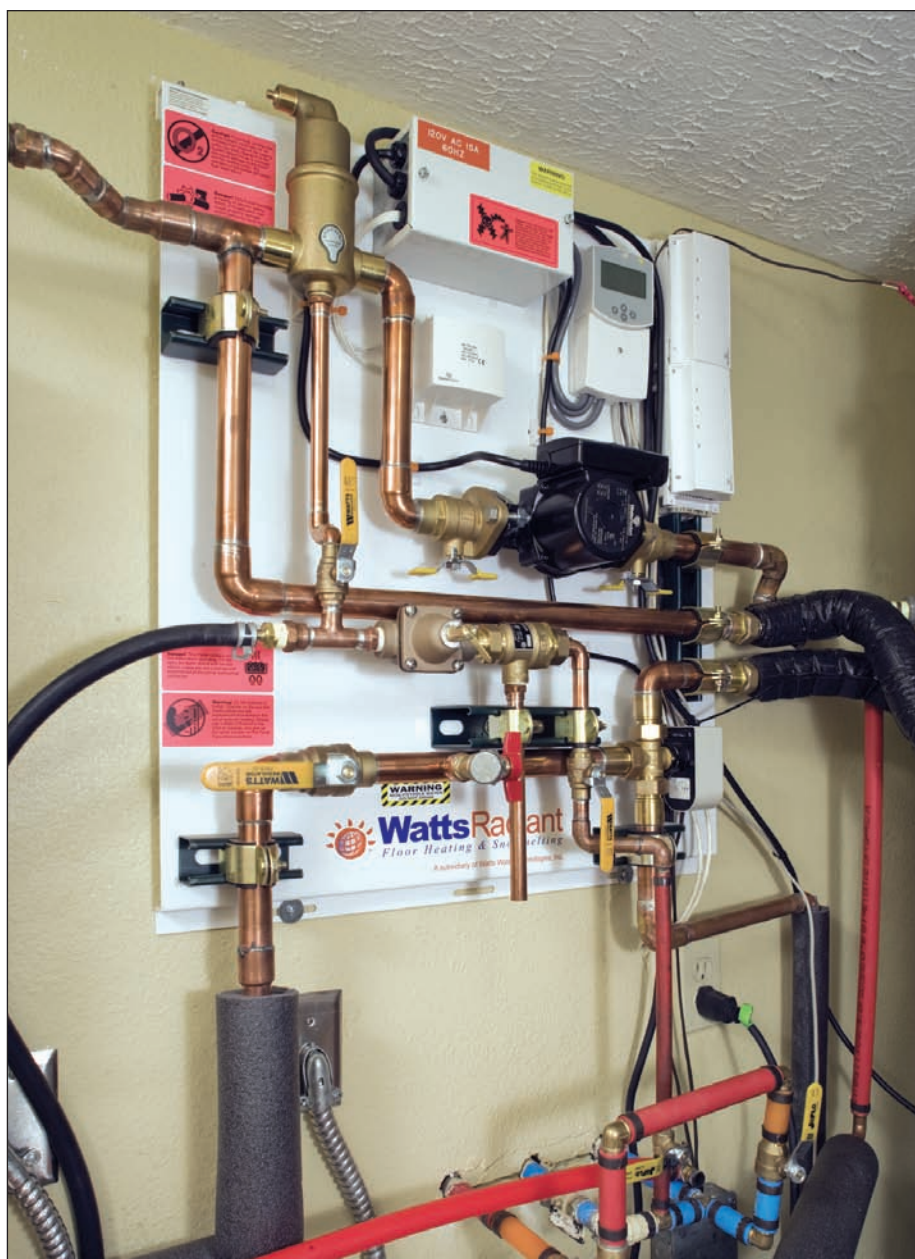
The Watts Radiant solar HydroControl panel incorporates a Caleffi Hydronic Controls solar pump station and stainless steel SolarFlex tubing to transport high-temp fluids from the panel to the indirect water heater.
