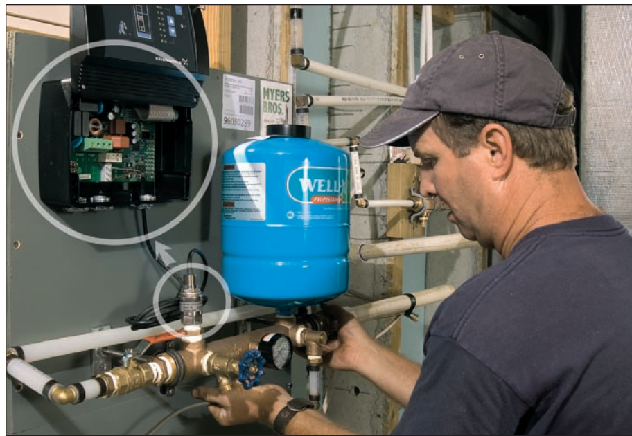
The pressure transducer maintains constant pressure by giving the controller a pressure signal that's used to increase or decrease the speed of the pump to sustain a constant, preset pressure in the 3,000 to 10,700 rpm range for gradual build-up or slowing-down of the motor for continuous maintenance of a desired pressure.
