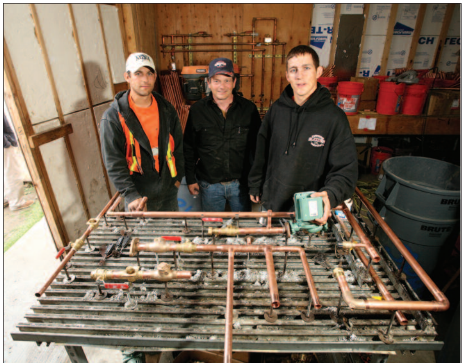
At one of Slayden's jobsite prefab assembly stations, Al Morlan (center) poses proudly with his two sons, Allen Jr. (left) and Joshua (right).
