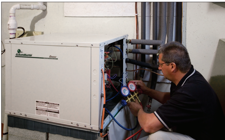
Dave Waltermire prepares to connect to the ClimateMaster's refrigerant ports for routine check of system performance.
