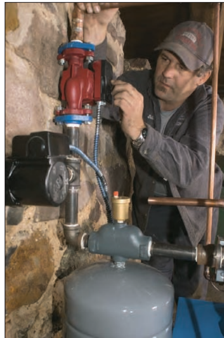
Haldeman technician Bill Aller makes an adjustment to a Grundfos three-speed SuperBrute circulator.
