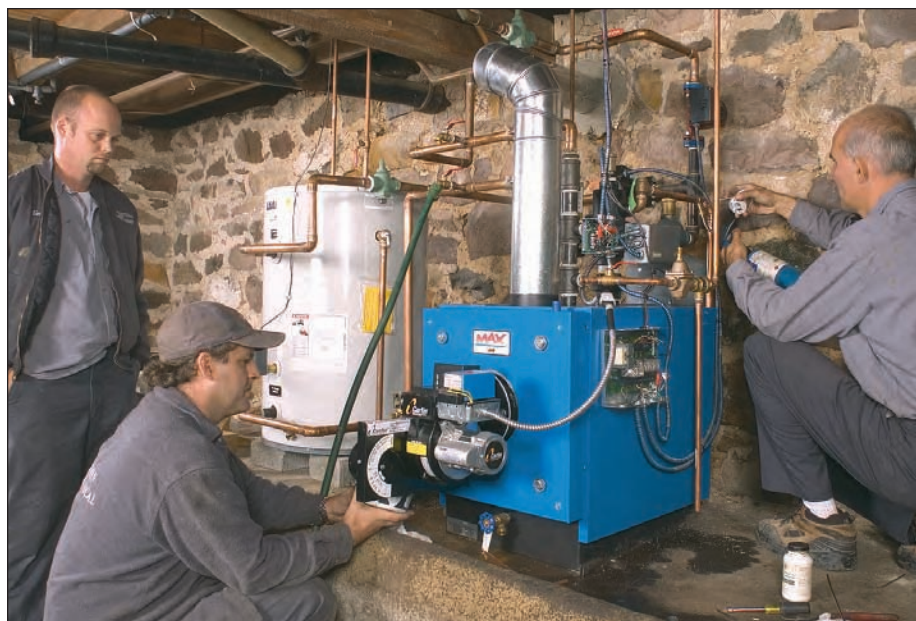
Haldeman technicians (from left to right) Gary Forry, Bill Aller and Tavi Nistor, complete the Laars Max boiler and indirect water heater installation.
