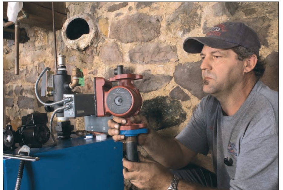
Bill Aller, hydronic technician, installs a Grundfos three-speed SuperBrute circulator.
