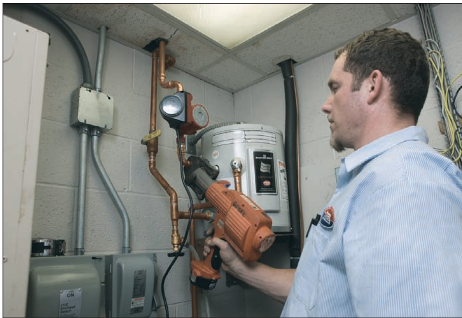
Jason Radesic, Geisel's plumbing service manager, installs a hot water recirculation system with a compact water heater at a Norfolk Southern Railroad facility.
