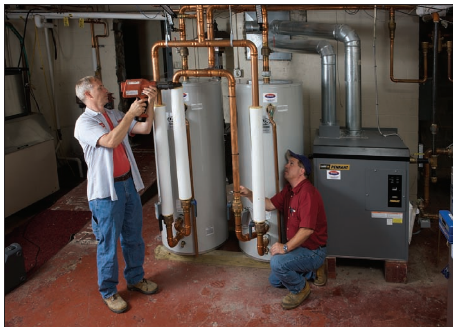
Tracy Ellan (r), plumbing manager for Geisel, oversees a solderless ProPress connection while installing a gas Pennant boiler for a country club client.
