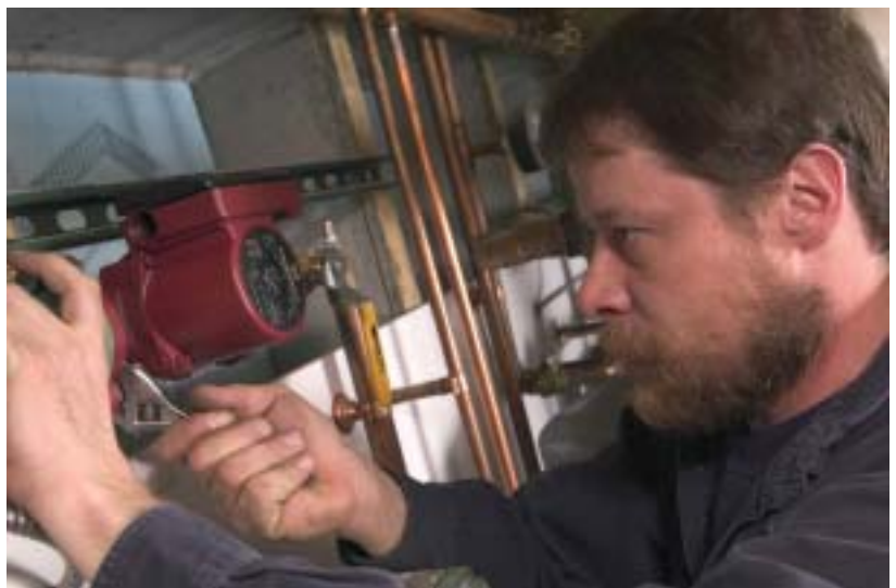
Bob Sieger installing.
