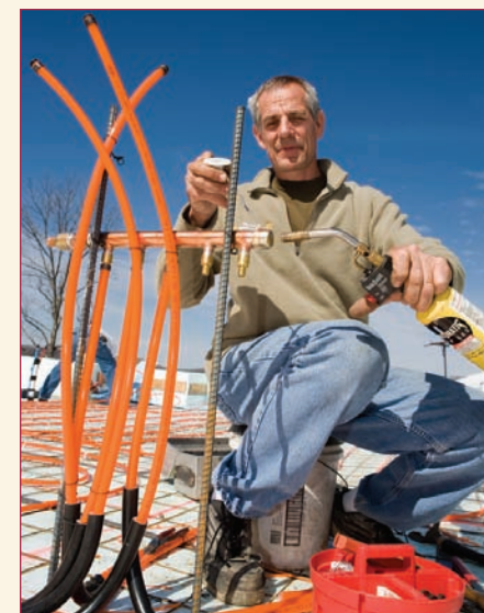
Hot rod roughs in a radiant manifold.
