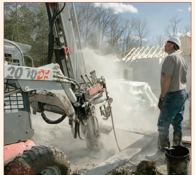
A different kind of Texas tea: geothermal drilling.
