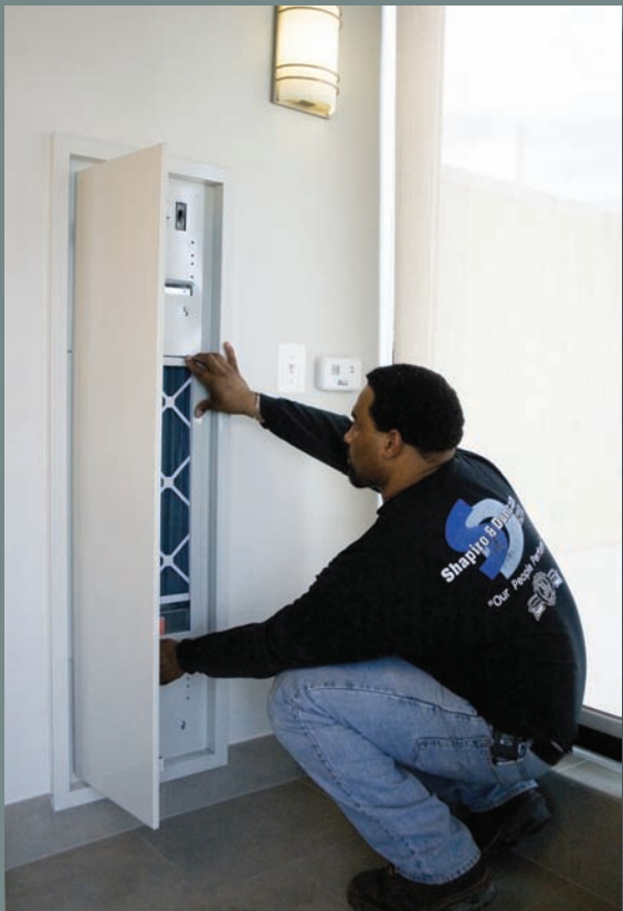
A ClimateMaster vertical stack unit is discreetly mounted within a condominium unit's main living area.
