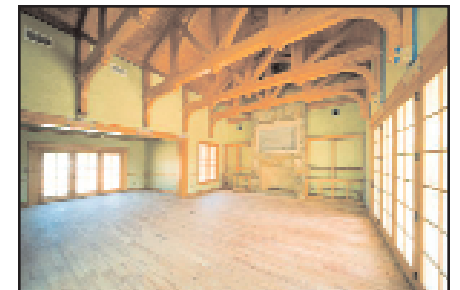
The attention to detail in the game room of the luxurious home is matched by the unseen radiant heating system.
