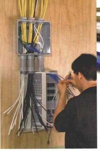
right, facing page). Each pair is capable of a separate function, such as a phone, fax or computer-network link. We don't install regular cat 5 anymore, preferring the broader bandwidth available with cat 5e *(e* for *enhanced)* cable. Cat 5e costs only about \$9 more per 1000 ft. than does cat 5, and it dramatically increases bandwidth. Cat 5 and cat 5e each cost more than twice what bell wire does. Although that sounds like a lot, the difference amounts to maybe \$50 for a house.
