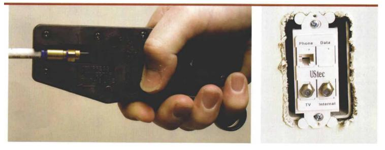
**F-connectors terminate RG 6 cable.** Having seen a 27-in. TV dangling from one, the author prefers the F-connectors made by Augat (Thomas & Betts; www.tnb.com). These connectors require an Augat IT1000 tool, which costs about \$60 but does the entire job from stripping the cable to crimping the F-connector.
