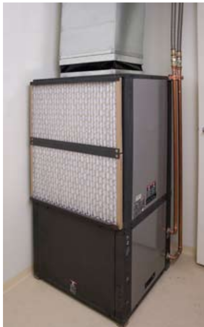
Water-source heat pump featuring R-410A refrigerant with a scroll compressor.
