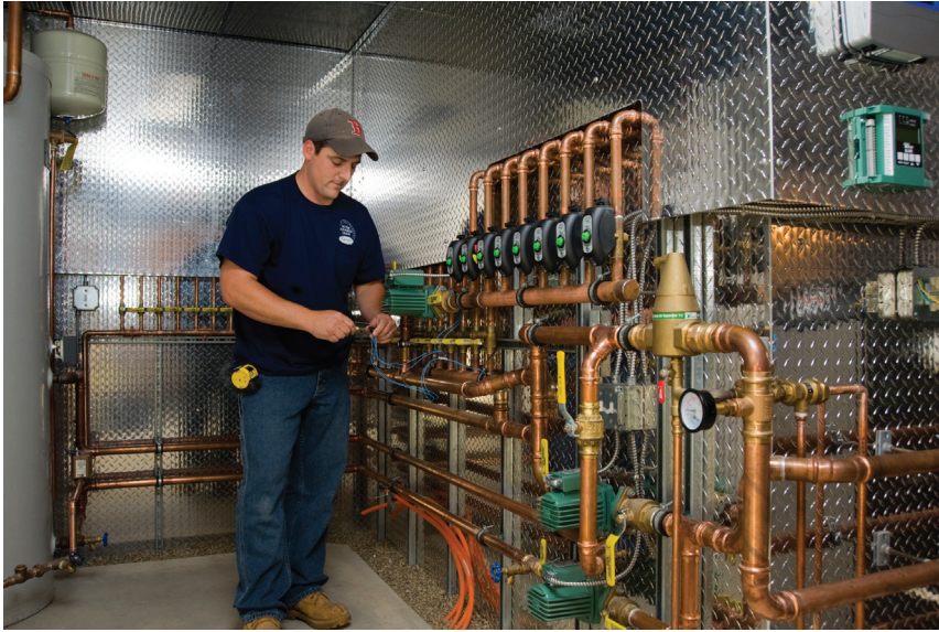
A technician completes the wiring for a light-commercial variable-speed-pump installation.
