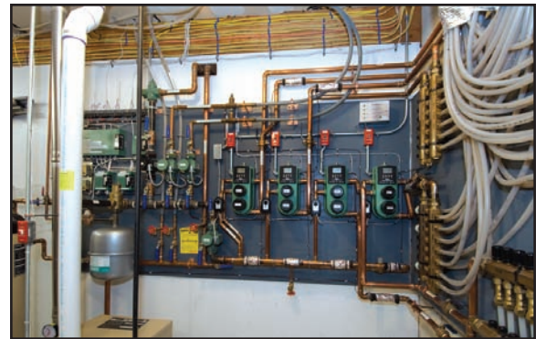
Taco RMBs have just four pipe connections, are quick and easy to install, and save space on mechanical boards. Taber described installing and wiring the RMBs as “so simple. Very easy to lay-out, plumb and wire.”
