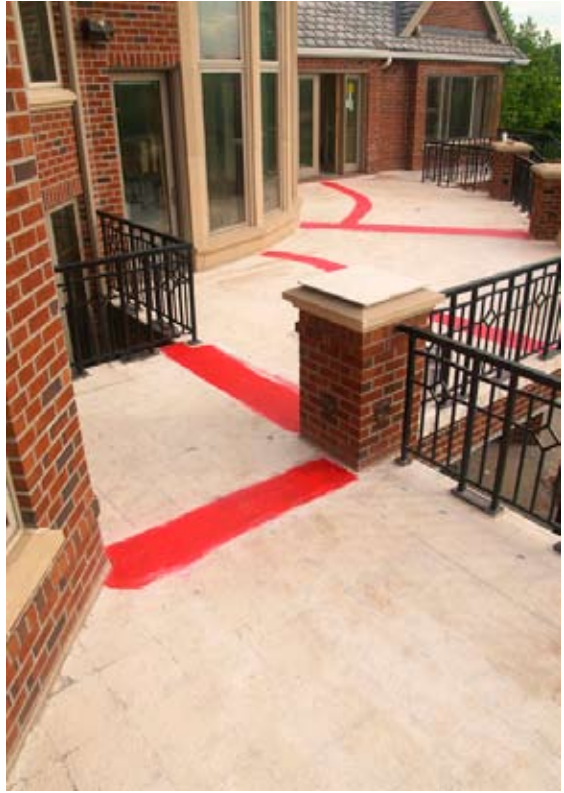
Preparing the deck to receive the snow melt cables included treatment with Custom Building Products' RedGuard® waterproofing and crack prevention membrane.
