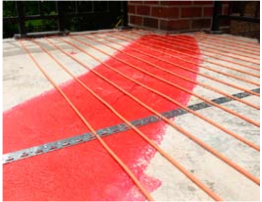
One circuit of the radiant heat/snowmelt cable system is complete.
