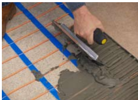
Installing SunTouch ProMelt mat under an exterior tile floor.
