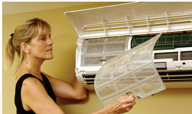
Indoor evaporator unit filters are typically easy to access, remove, and clean. Just behind the removed filter is an indoor air quality (IAQ) filter cartridge.
