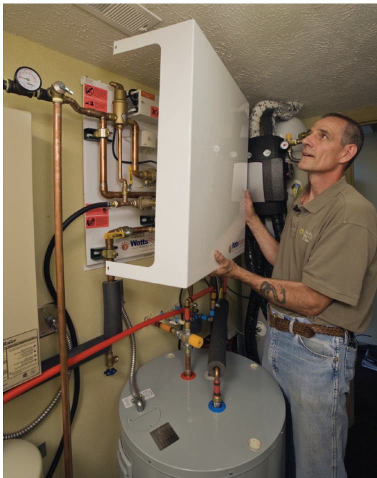
Watts Radiant supplied the Habitat house with a solar HydroControl panel, radiant tubing, radiant heat manifolds and aluminum dispersion plates.
