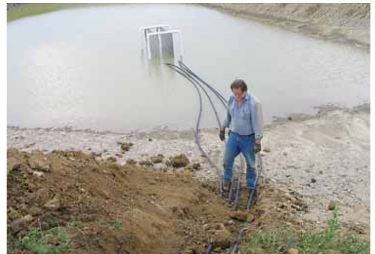
If a suitable body of water is nearby, lake plate heat exchangers are an excellent way to harvest thermal energy for geothermal systems.
