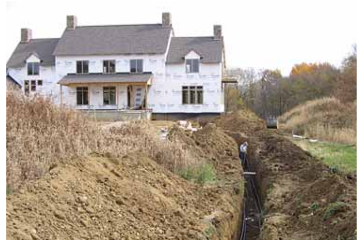
Deep geothermal bore-hole supply and return lines must be trenched below the frost line.
