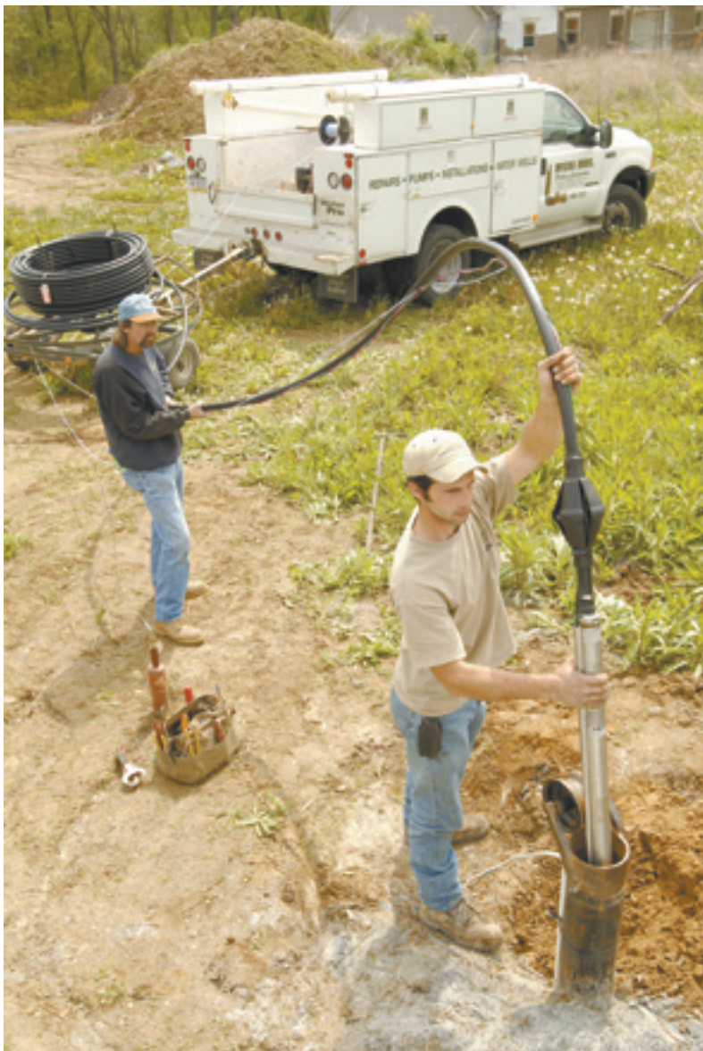
Tom Sherk lowers the pump into the well with assistance from Robert Hummel.
