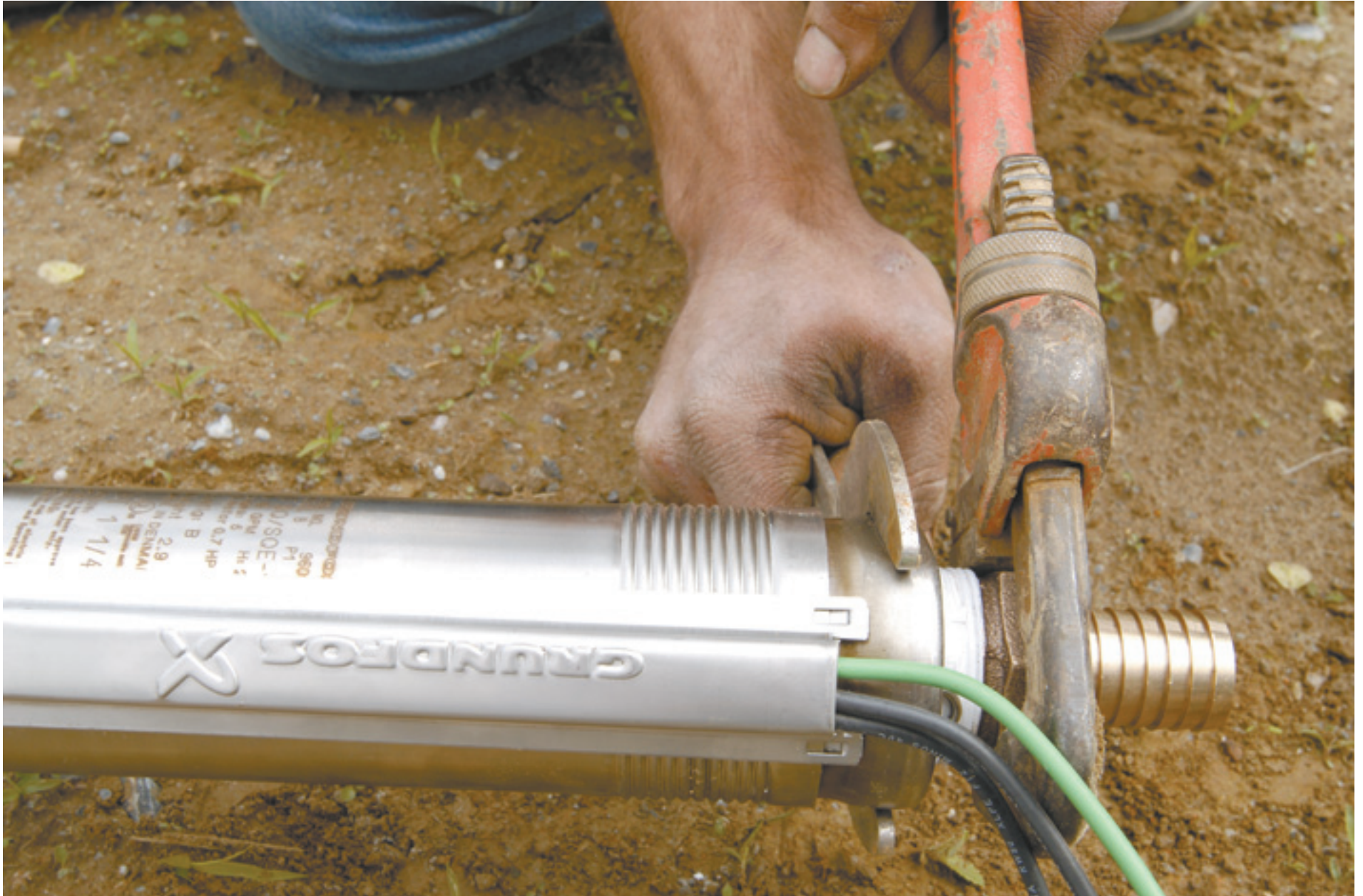
Preparing the pump for installation.
