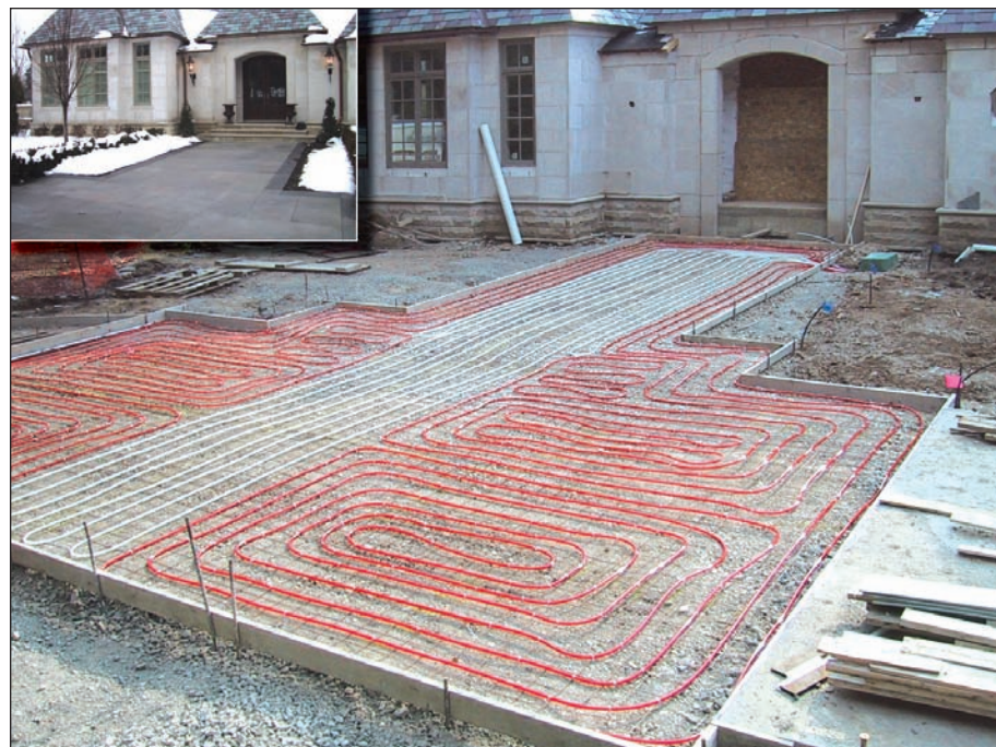
Hydronic snowmelting systems find a host of applications such as this popular means of clearing snow and ice from entryways at private homes. Radiant snowmelting systems clear snow completely, leaving a clean, dry and safe walking surface.
