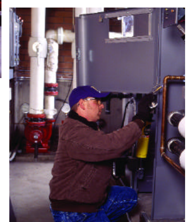
A McKinstry contractor solders a connection to the Rheos boiler.
