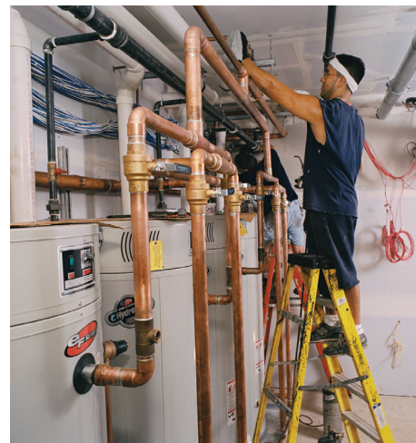
An eF water heater installation in a New Jersey hotel.
