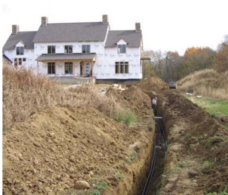
Geothermal lines are trenched from a lake loop into a home.
