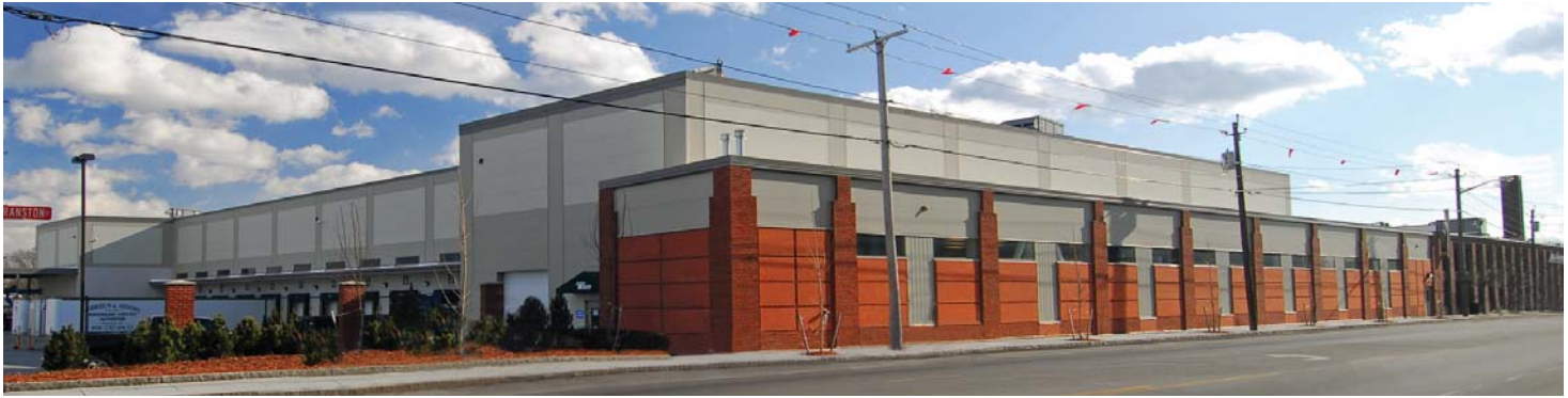
Taco's new, LEED-certified warehouse in Cranston, RI.
