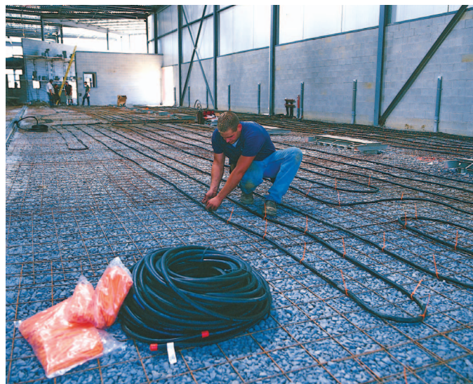
⤴ Techs tie down EPDM radiant-heat tubing in the area where auto mechanics work at the Volkswagen dealership in York, PA.
