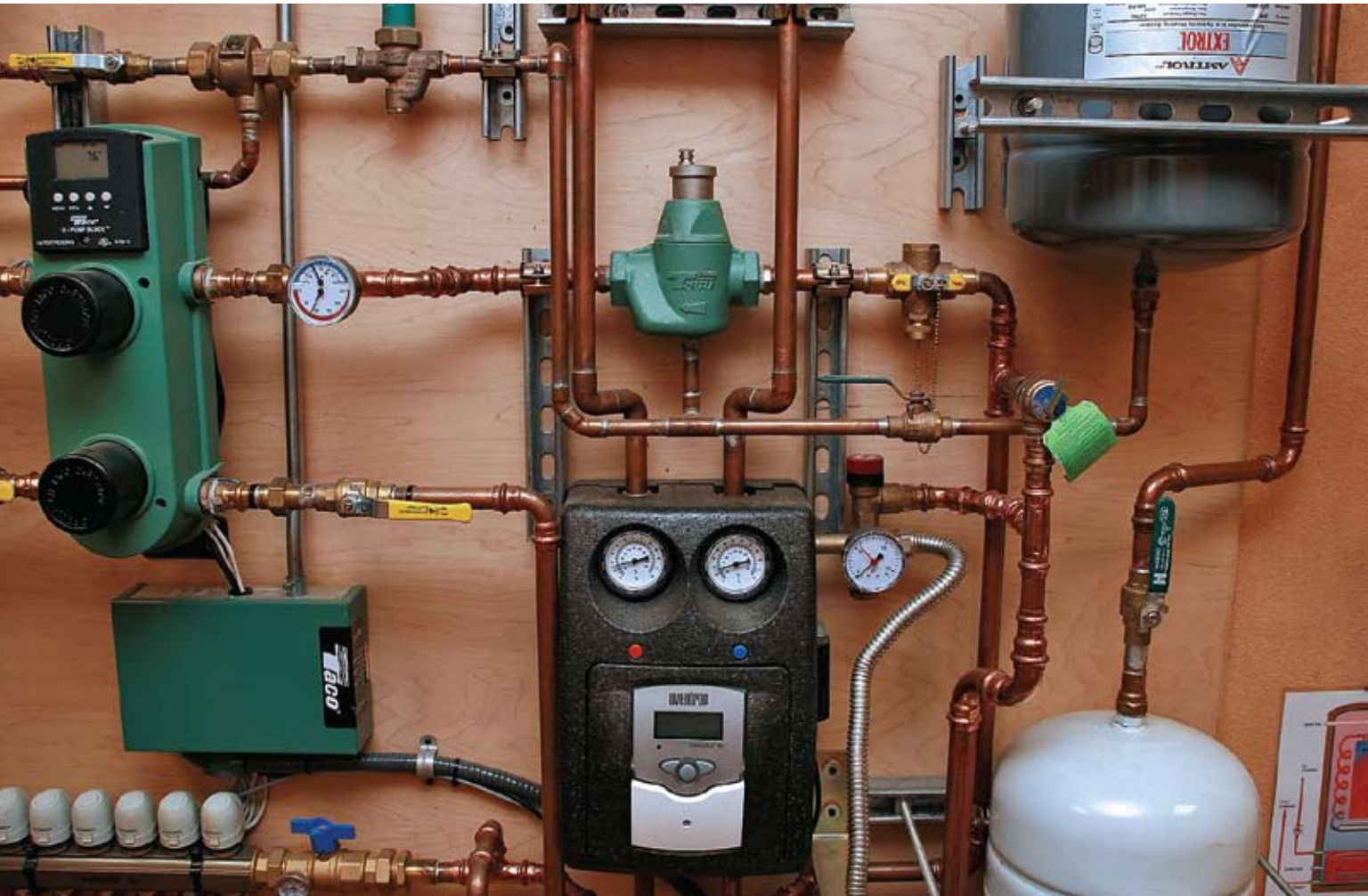
The controls and components board for the solar thermal system at Humboldt State's Campus Center for Appropriate Technology, including the pump block, pumping station and thermal actuators.
