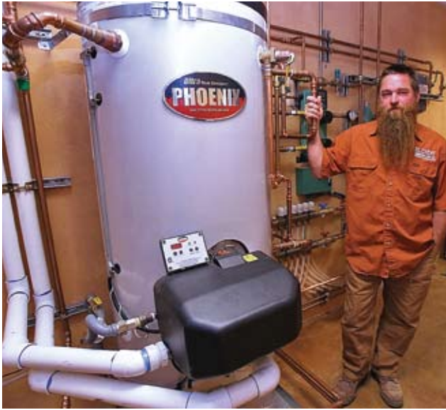
Stephen Bohner of Alchemy Construction with the newly installed solar water heater, which provides hot water storage and boiler back-up to CCAT's solar thermal space-heating and domestic hot water systems.
