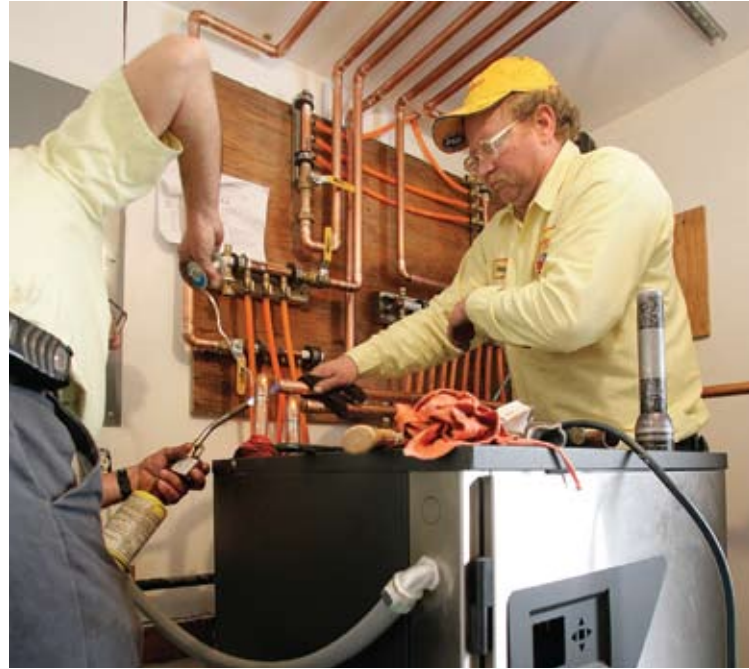
Gabrilson's Dave Pollitz (left), senior service technician, is soldering the supply line to the Carrier geothermal system; he is assisted by Denny Hesse, senior installation mechanic.
