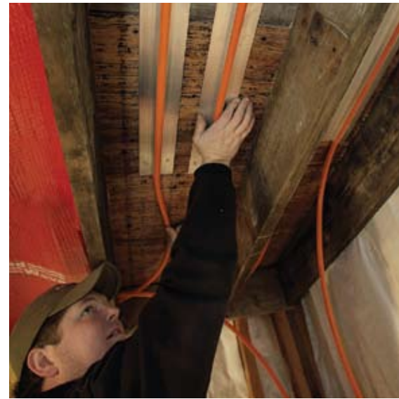
Left photo: Chad Pregracke (middle) takes a moment at the project's completion with Gabrilson's Dave Pollitz (left) and Denny Hesse (right). Right photo: Installation of the PEX tubing under the mezzanine area included extruded aluminum plates for optimal heat transfer.
