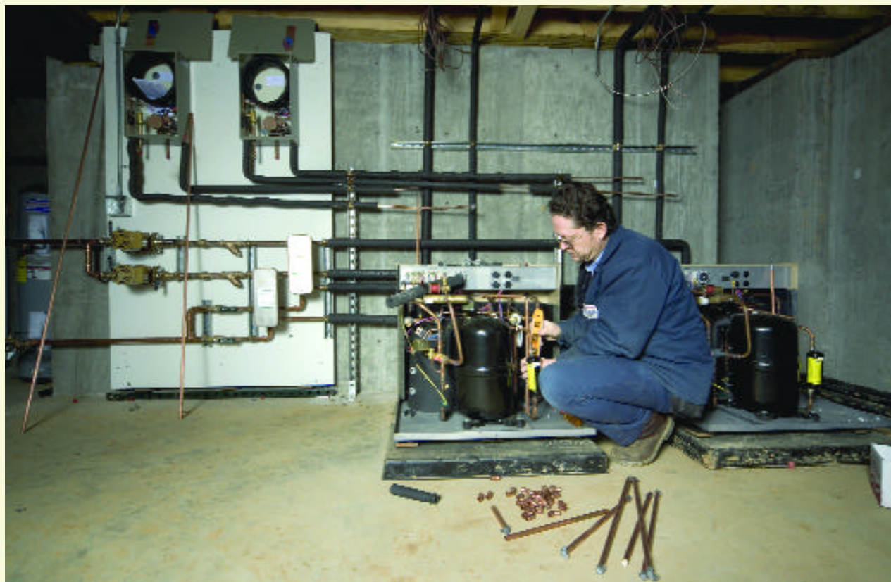
Dave Yeager, a tech with Oren Atchley Co. Inc., makes connections between the geothermal heat pumps and the radiant heat system.
