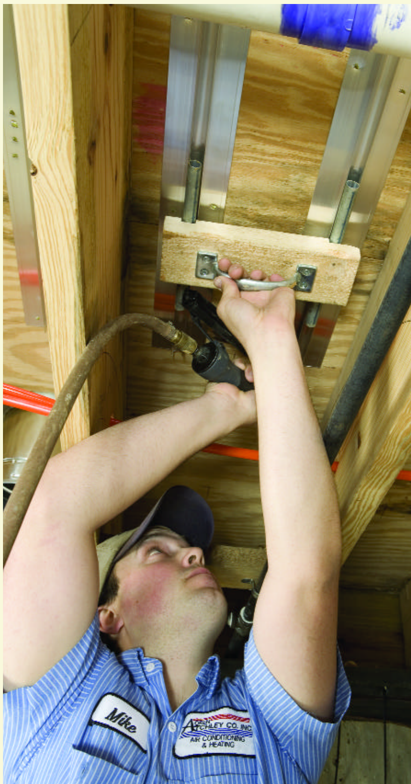
Mike Yarbrough puts the finishing touches on a radiant staple-up system.
