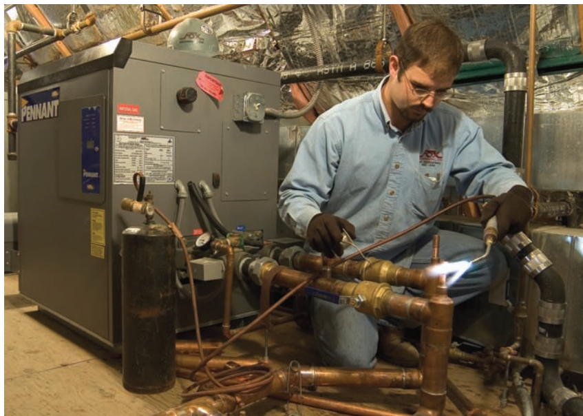
The attic mechanical room was truly a tight fit.
