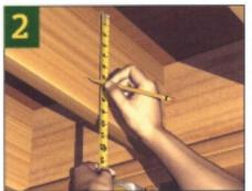
Measure and mark the floor joists to be bored. Before you bore engineered joists, consult the manufacturer.
