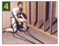
Begin the process of pulling tubing by walking a double length of it to the end of the first joist bay.
