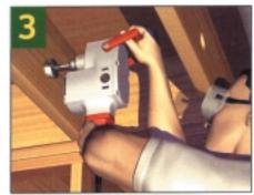
Bore the holes through the joists with a rightangle drill and a self-feeding bit. Position yourself under the drill and behind it. Maintain a firm stance with sound footing.
