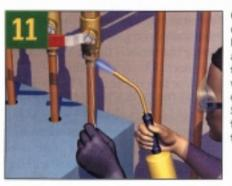
Cut the boiler's copper tubing to length, then clean and fit the parts together with valves and other components. Solder each joint from the bottom to the top.
