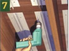
Begin PEX installation by fastening its aluminum channels to the floor deck using self-tapping sheetmetal screws driven by a cordless drill.
