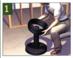
To prevent tubing from becoming tangled as it's installed, place the roll on a spooler.
