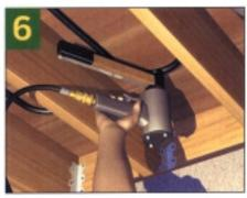
To fasten EPDM tubing quickly, you need to rent a staple gun with a specially shaped nose piece. Staple the tubing in the first jolst bay at 6-to 8-in. Intervals. Once fastened, pull the tubing for the next joist bay.
