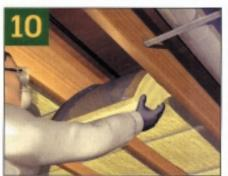
Once both types of tubing are installed, insulate below with fiberglass batts. Place the foil facing up, about 2 in. below the tubing. Support the insulation with pieces of wire or manufactured supports.
