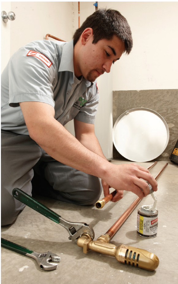
Technician Derek Sanderson assembles a leak protection system for the water heater.
