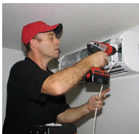
Technician Nelson Vokey installs an air handler.
