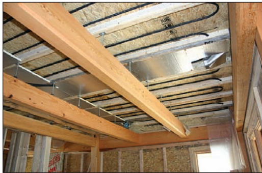
Ciardelli made extensive use of Watts Radiant's Onix EPDM rubber staple-up tubing in the radiant-floor heating system of its new headquarters.
