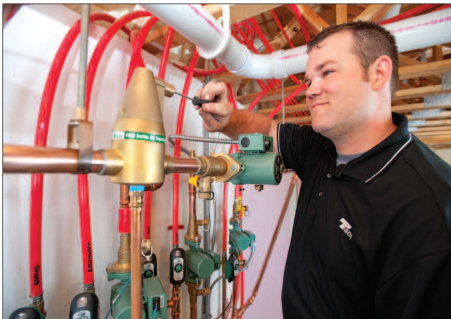
Before purging a newly-installed system, Aune verifies that the air separator is closed.
