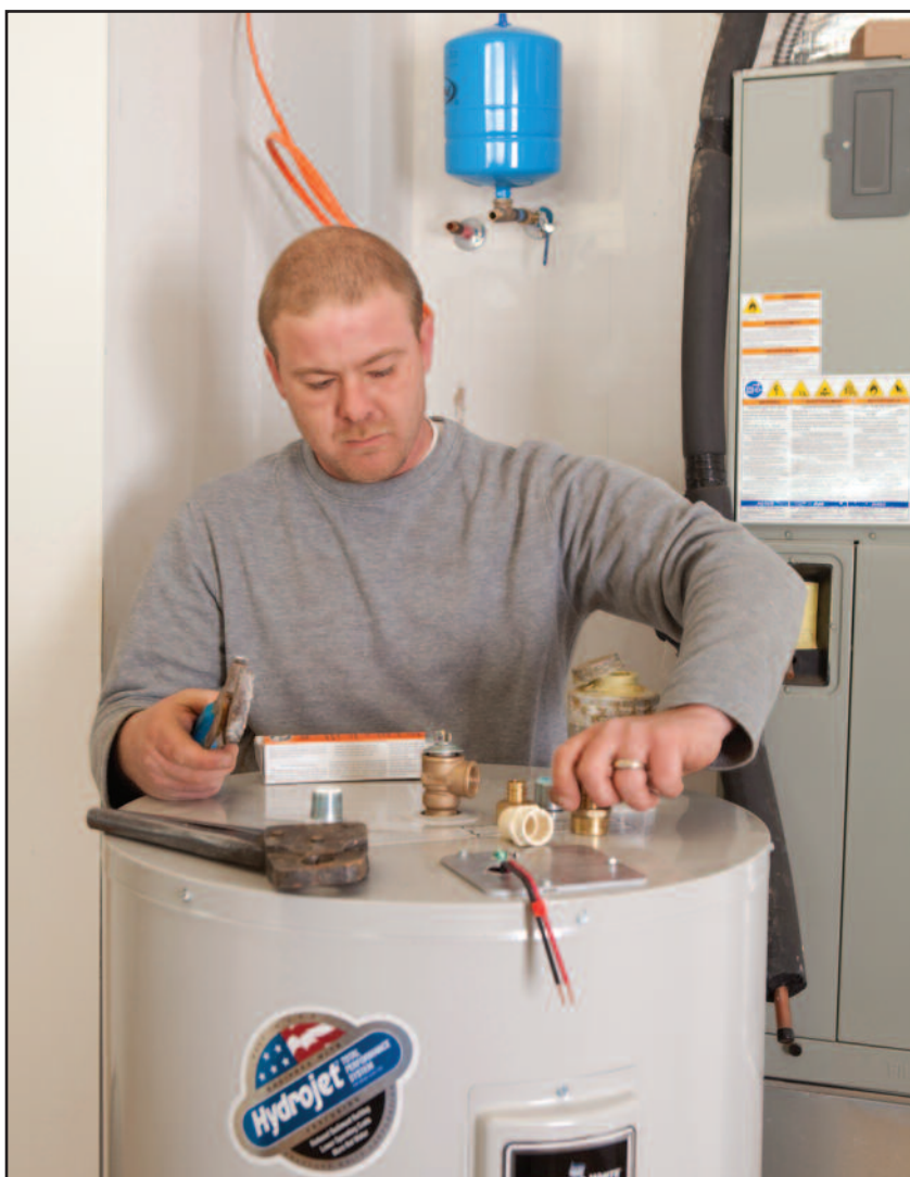
Plumber Derrick McGough installs a water heater.
