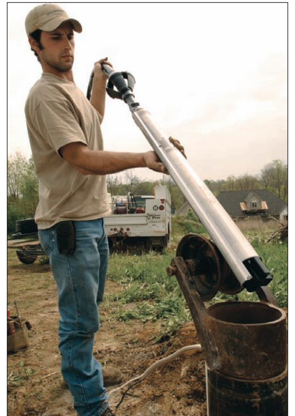
Big power, small package: The Grundfos SQE submersible pump with VFD technology provides all the water the homeowners need for their 5,000-sq.-ft. home that eventually will feature six bathrooms.
