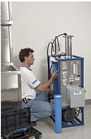
The amount of storage space available for the equipment will determine the size of the RO and storage tank. Ideally, production or output of the RO system should be about 1.25 times (or greater) the mist unit's consumption.
