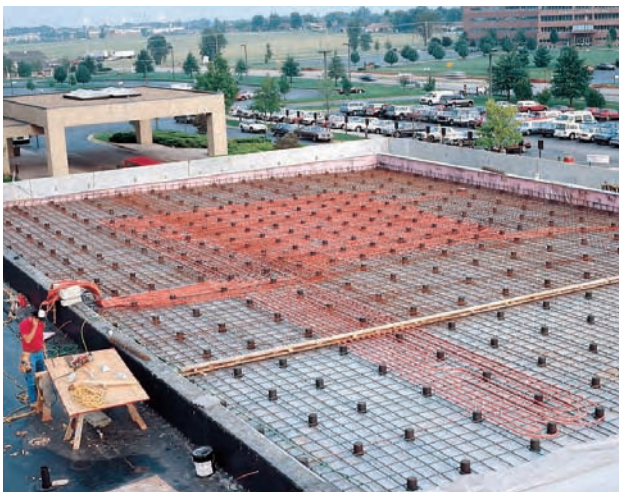
PEX installed at this hospital heliport helps to melt snow.
