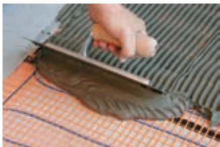
Thin-set mortar can be troweled directly over the electric radiant heat mat.
