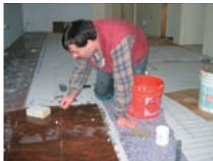
Pejic installs stone tile over the floor warming mat.
