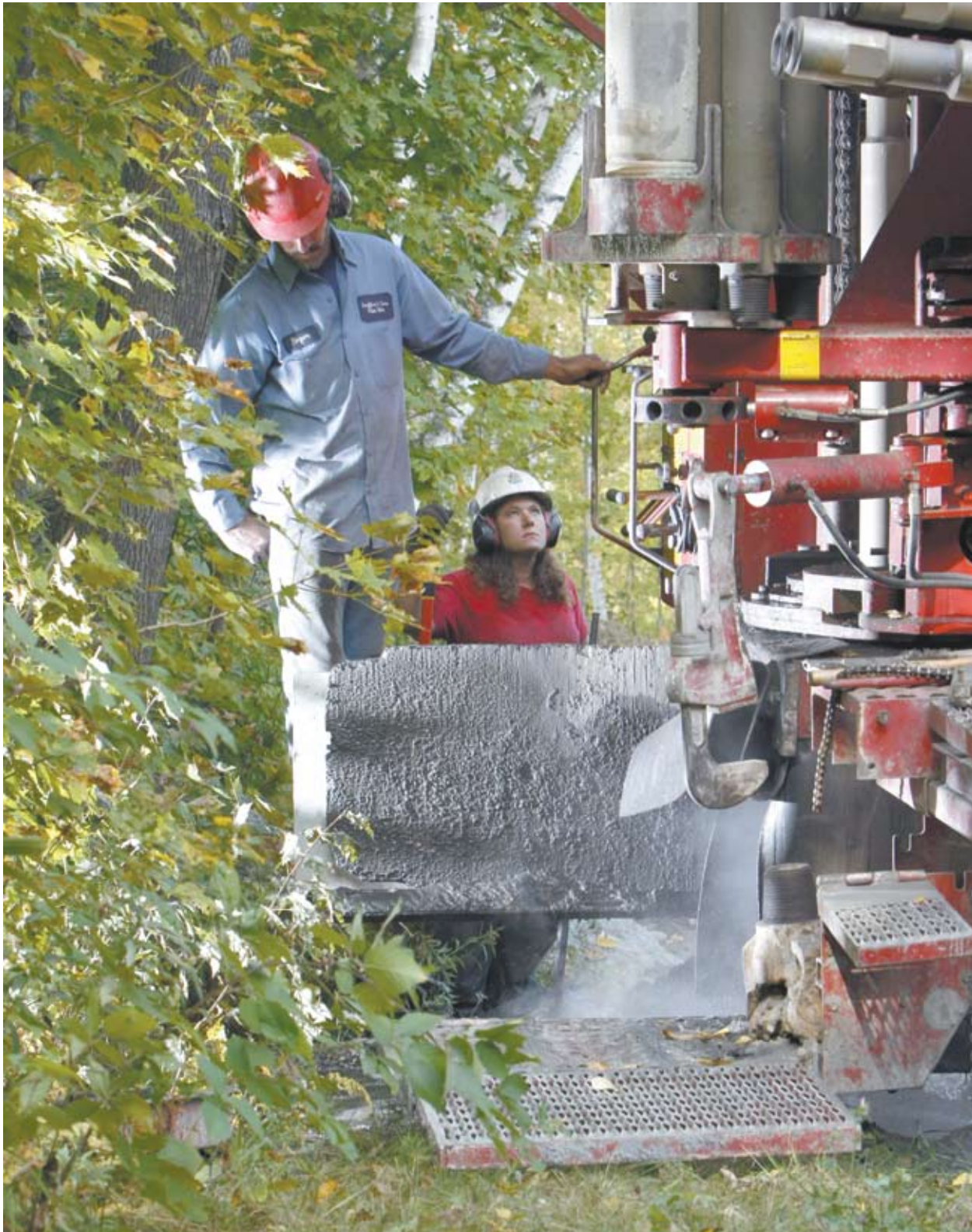
Roger “Farmboy” Gagnon and Melissa “Diesel” Mullen drilling a 12-inch bore to set 8-inch casing.
