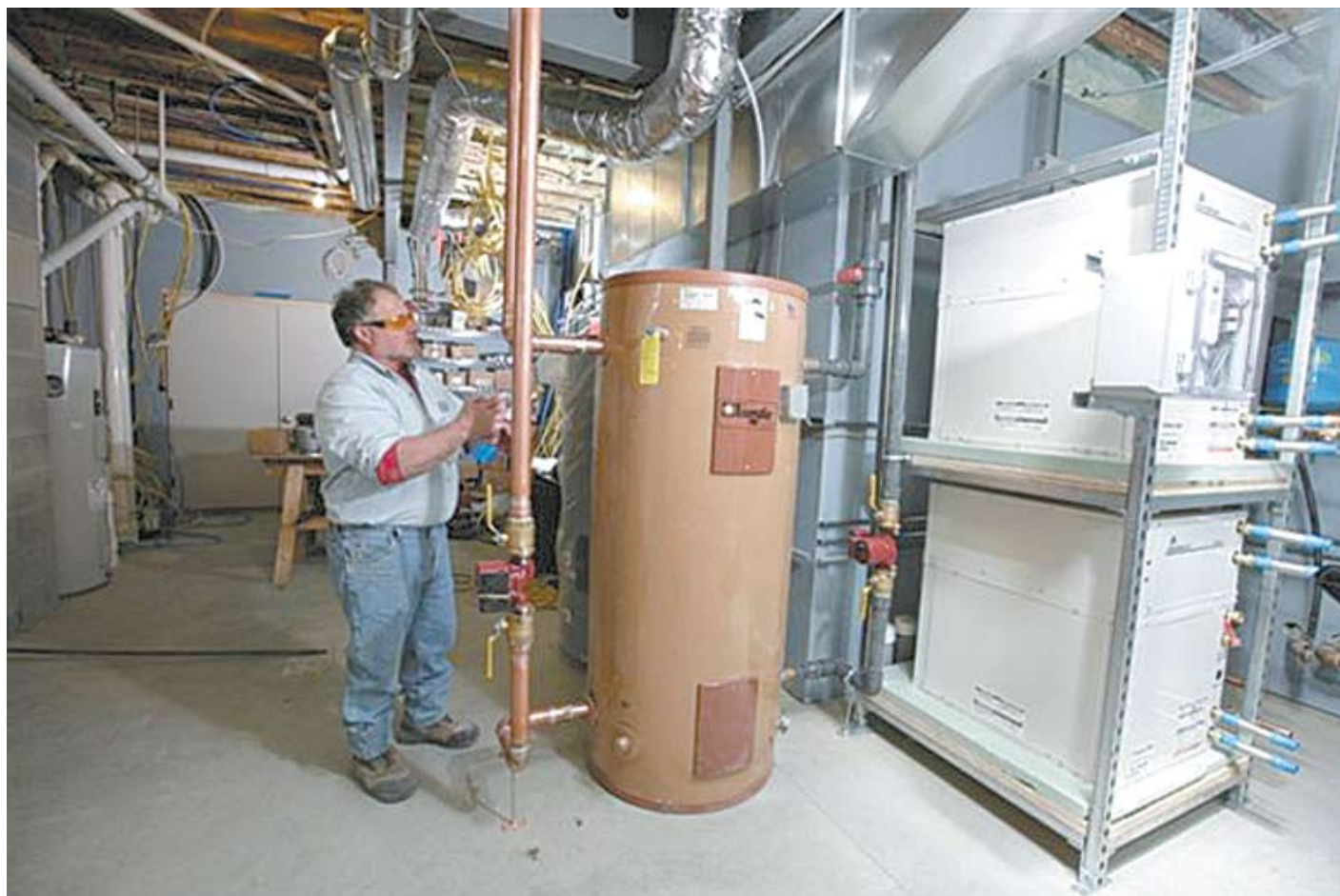
Dean Muniz installs a geothermal buffer tank.
