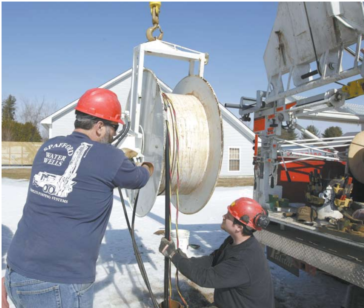
Jeff Willams and Ian “Cracker” Labounty pulling a very deep pump.
