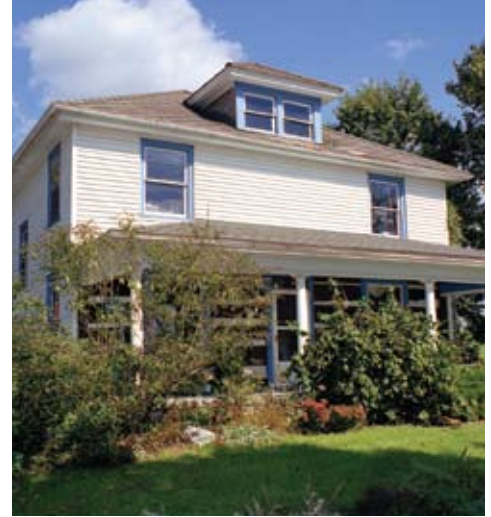
The Martin home undergoes its first-ever major renovation.
