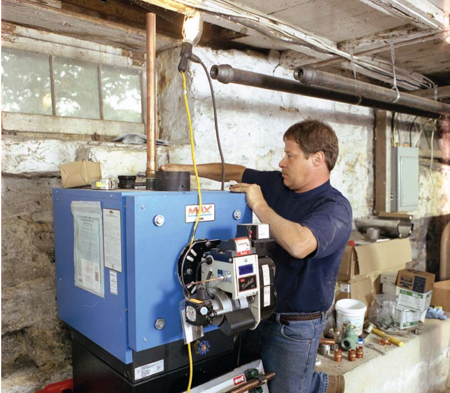
Bob Seiger, senior technician, installs the new boiler's vent stack.
